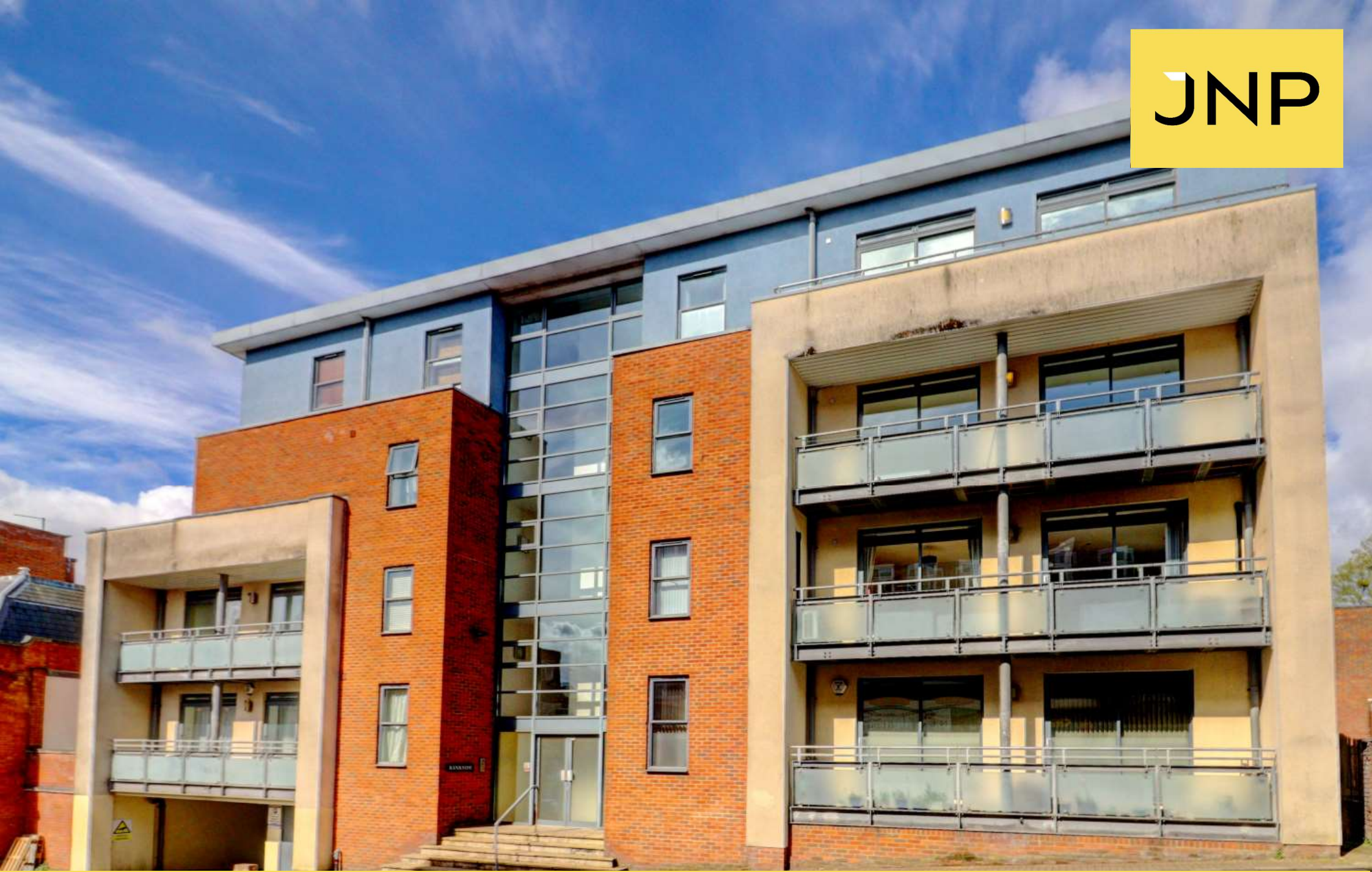
Flat 16 Bankside, Corporation Street, High Wycombe, Buckinghamshire, HP13 6TA Asking price £285,000 Leasehold
